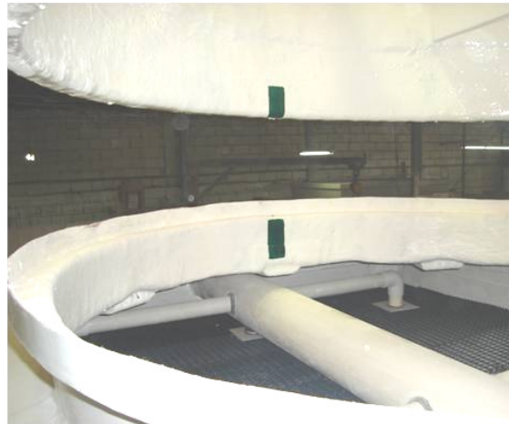
Figure A-14: Fan Duct Alignment
