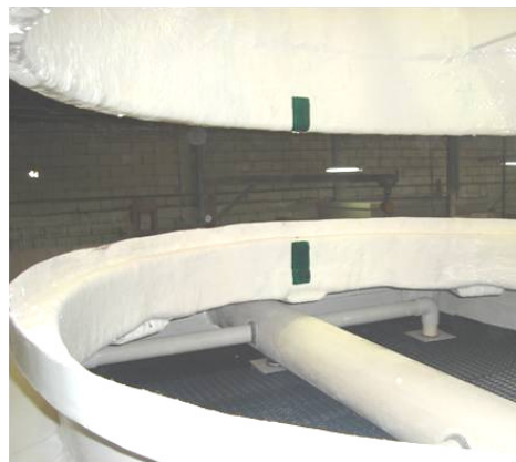
Figure A-40: Fan Duct alignment
