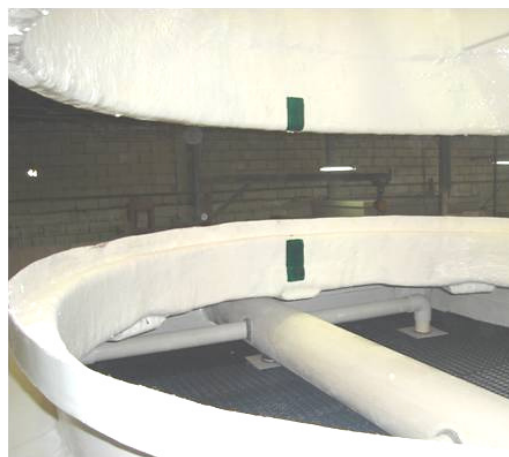
Figure A-37: Fan Adaptor Alignment
