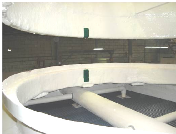
Figure A-8: Fan Duct Alignment
