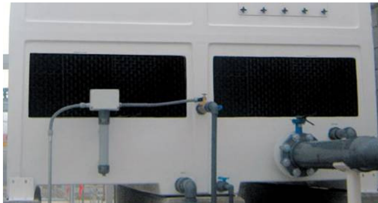
Figure A-53: Water level control system
